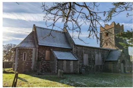
North Side of Church from Sanctuary Side
