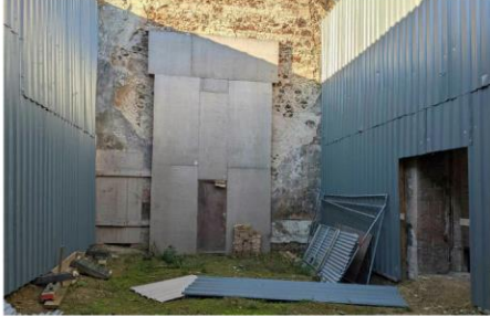
Looking West in the Nave
