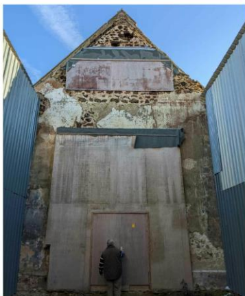
Looking at Chancel Wall from Nave
