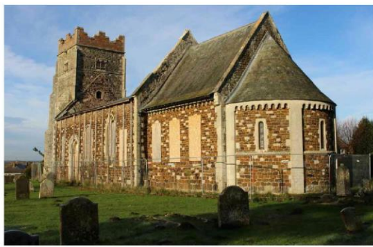
South Side of Church from Sanctuary Side.
